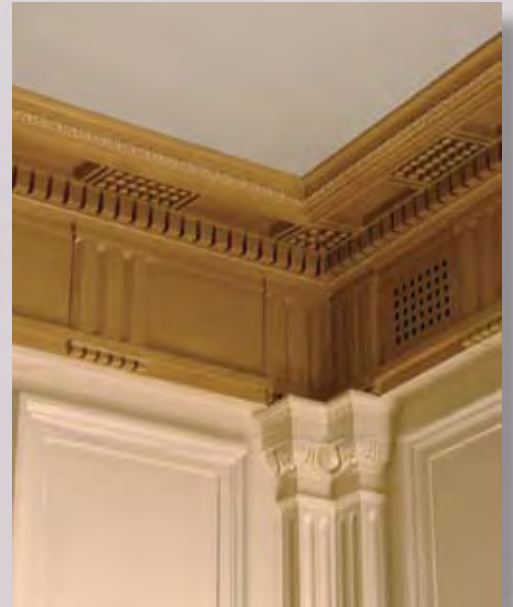
Custom frieze, corner pilaster and panel moulding.
