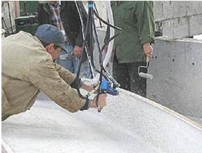
Figure 5: Hand spraying Zoho Stone's GFRC
