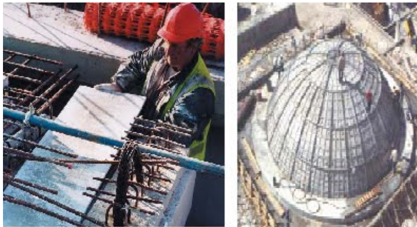
Figure 11: Zoho Stone's GFRC Permanent Form Work
